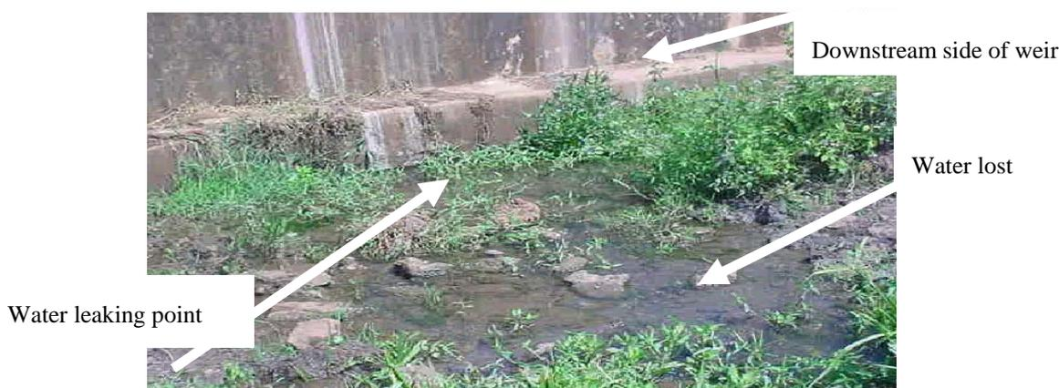
Figure 4: Leakage on Geray River Diversion
