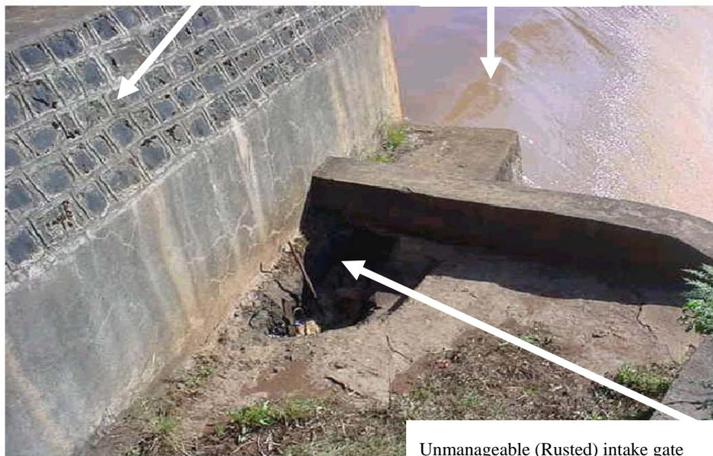
**Figure 6: An intake gate of Fetam Diversion**
